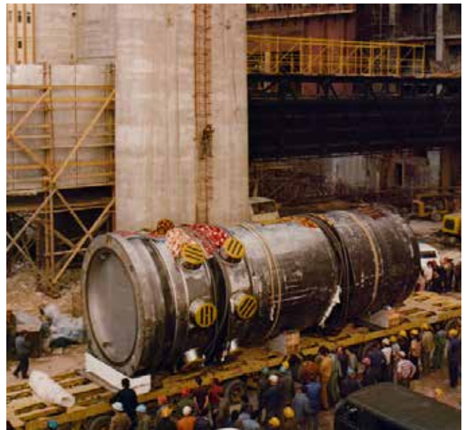
Figure 1: The reactor pressure vessel with the nozzle ends
